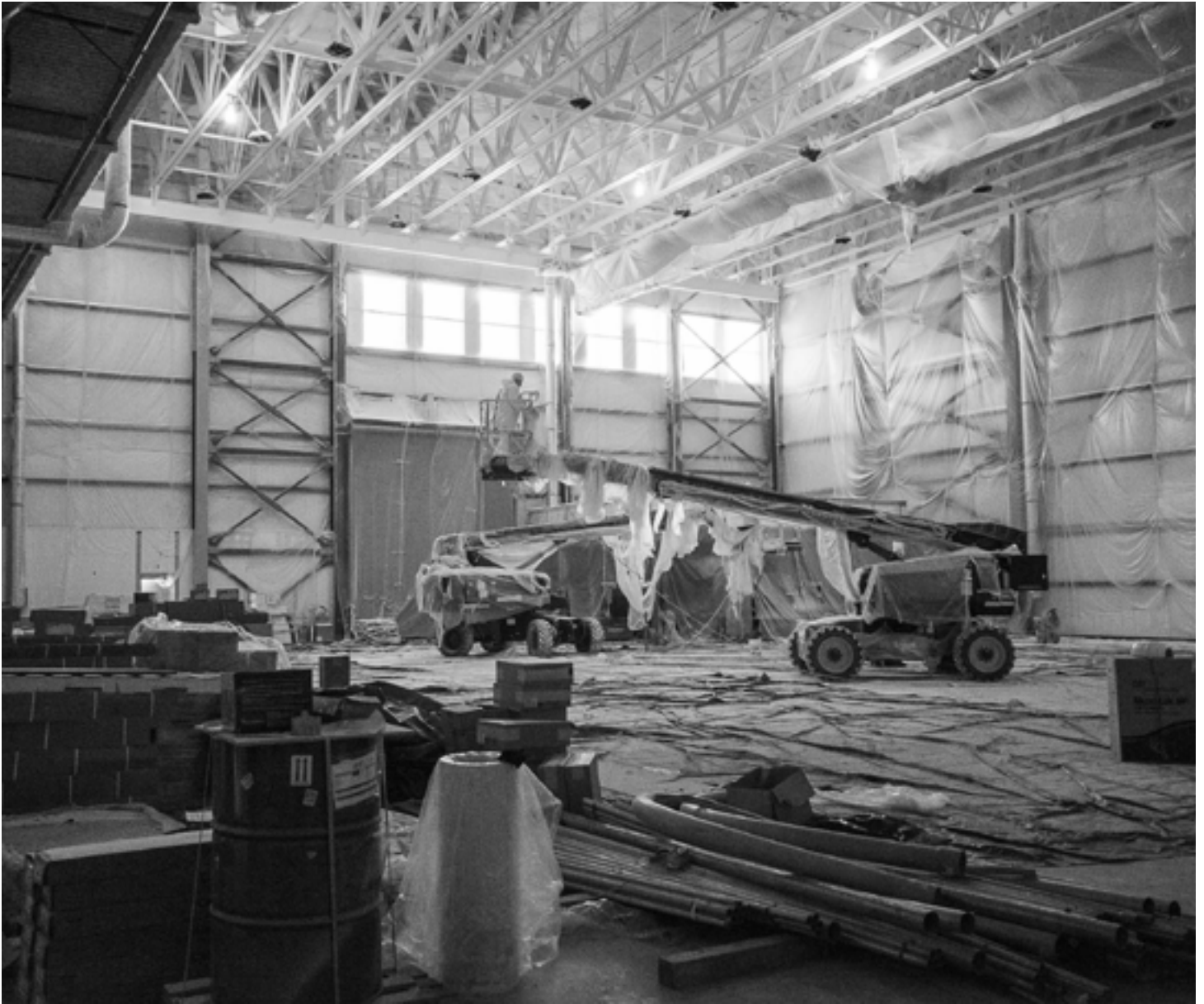
IMAGE 06. Simulator bay under construction.
